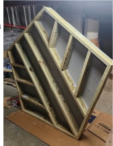
Blind Floor Framing
